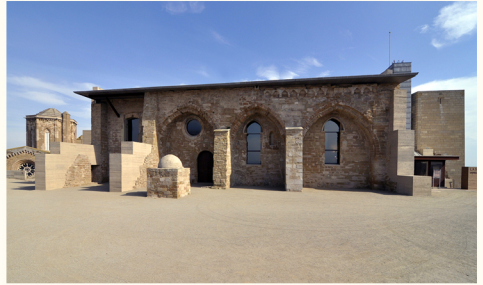
North façade of the former Corts Hall
